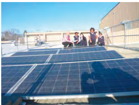
Figure 1. Teacher with students with the rooftop solar panels
